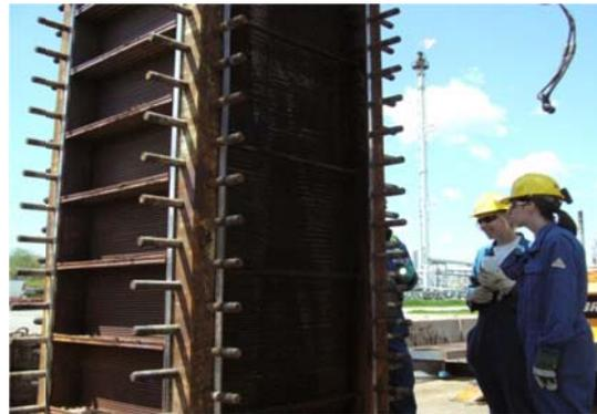
Figure 3 Alfa-Laval Compabloc Heat exchanger: CC 106A. Inspection prior to the cleaning
