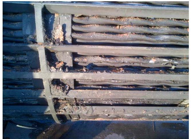
Figure 1: Exchanger Prior to cleaning
