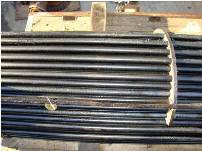
Fig. 3 Tube bundle removed from warm exchanger, nearly no fouling (feed on the shell side)
