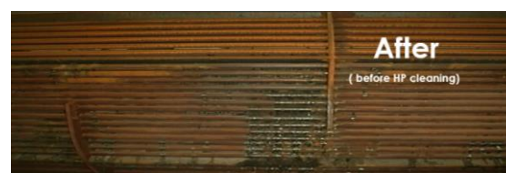
Fig. 12. Popcorn pollution thermal cleaning (before HP cleaning).
