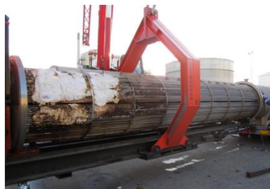
Fig. 16. Extraction of a bundle from its shell.
