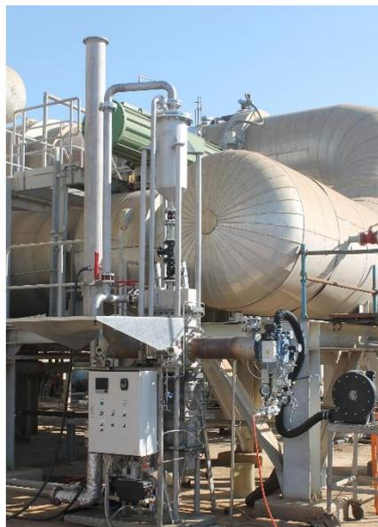
Figure 1. Pilot unit installed at one of the MSF distillers at the Sabiyah power plant.
