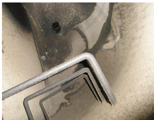
Fig. 9. Tower bottom—Deposits have been dissolved by ITW.
