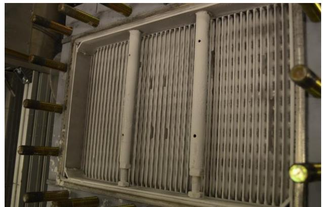
Fig. 5 Deposits formed on the heat exchanger plate pack after water-salt scaling.
