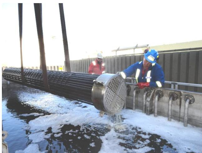
Fig. 3. A typical exchanger being removed from the ultrasonic bath for inspection and rinsing.
