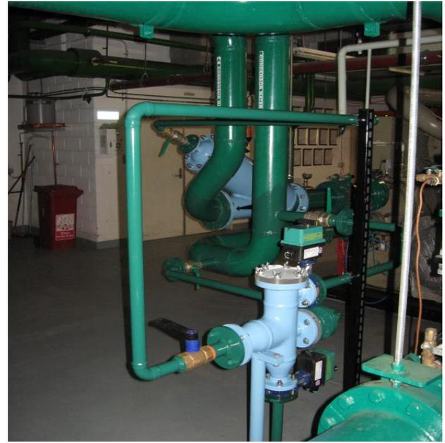
Fig. 3 The sponge ball ATCS installed in Case 1
