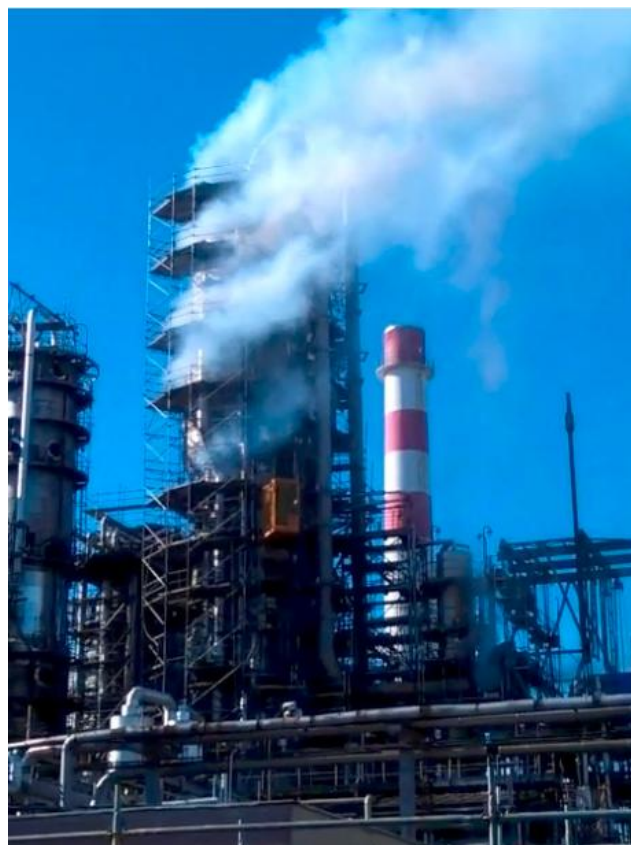
Fig. 1: Pyrophoric iron fire in a distillation column
