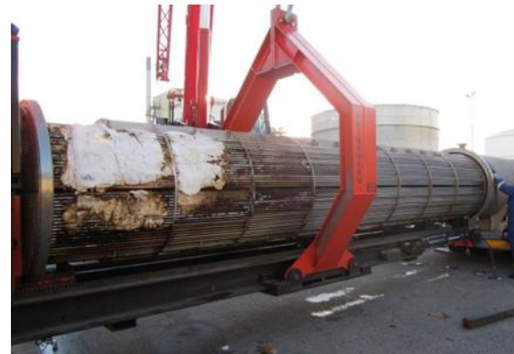
Fig. 16. Extraction of a bundle from its shell.
