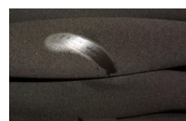
Fig. 7 Exchanger E-4 Shell Side Foulant
