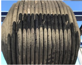
Fig. 12. E-1 Before - U-bend Close up
