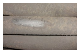
Fig. 6. Exchanger E-2 Shell Side Foulant
