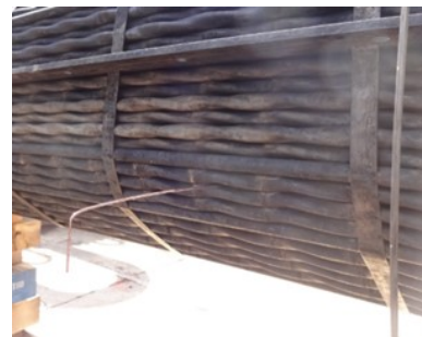
Fig. 4. Previous Cleaning Attempt. Shell Side fouling layer still observed after chemical cleaning in-place and HPWB. Debris still built up between the tubes as evidenced by the Dip Stick verification.
