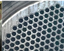
Fig. 17. E-4 After - Tube Side Cleaning
