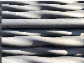
Fig. 11. E-1 After - Shell Side Close up
