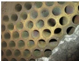
Fig. 16. E-4 Before - Tube Side Fouling
