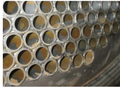
Fig. 3. Previous Cleaning Attempt. Tube Side fouling layer still observed after chemical cleaning in-place and HPWB.
