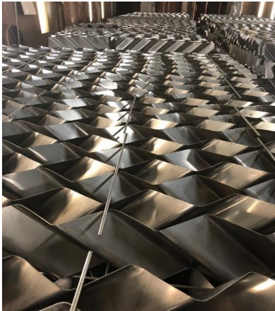
Fig. 14. Crude Unit Vacuum Column wash bed (316 SS) installed in July 2020.
