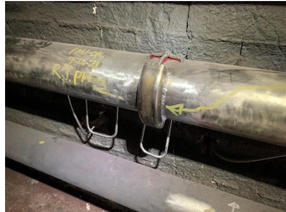
Fig. 15. Coker furnace pipe replaced with Minimox-treated pipe, upper pipe (347H SS) installed in October 2021.
