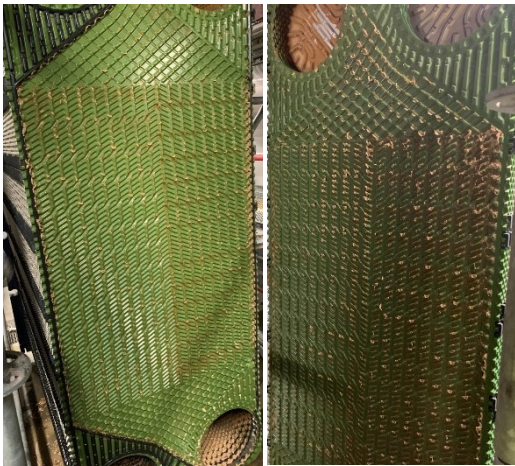
Fig. 12 – Fouling on the 2-layer coated channel.
