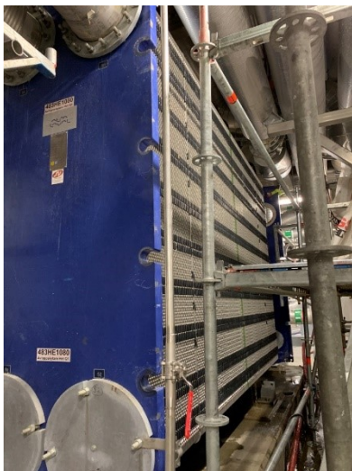
Fig. 1 - The WG350 GPHE (HE1080) with the coated plates at the customer site.
