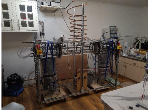
Figure 12. The vacuum boiler
