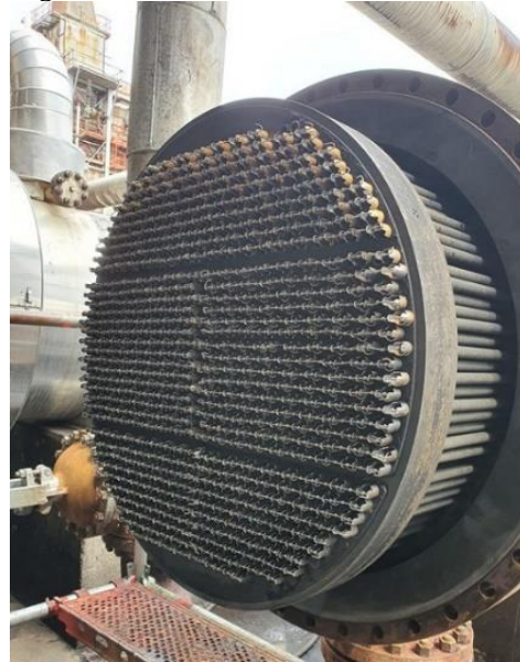
Figure 2 - Photo of the Spirelf® on a tube bundle
