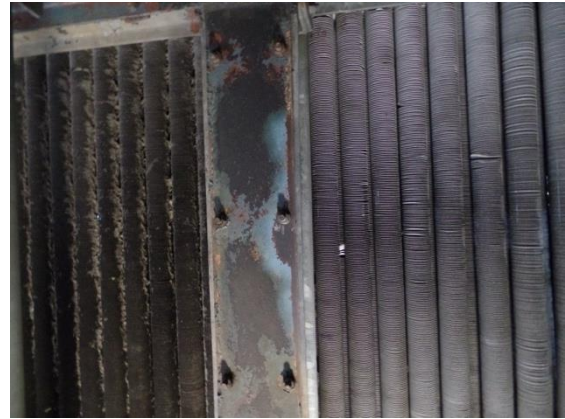
Figure 5: Adjacent dirty and cleaned bundles
